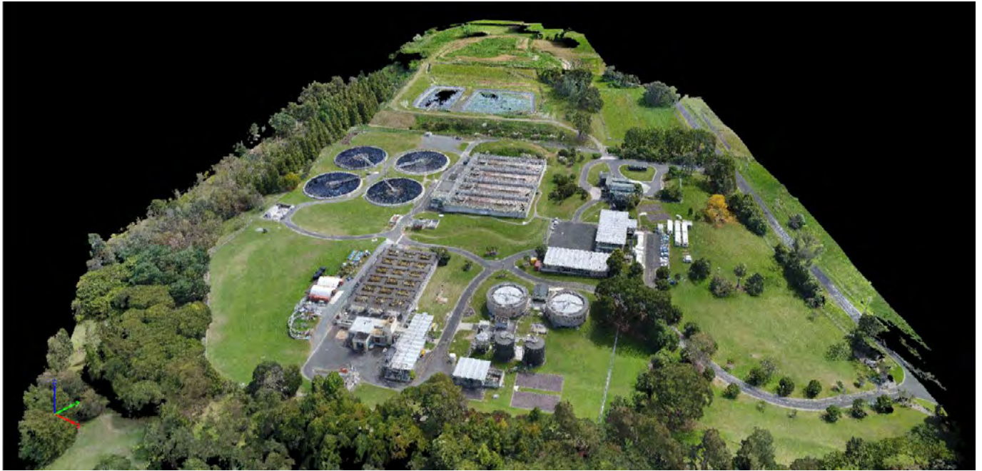
Figure 10: Pukete Wastewater Treatment Plant
